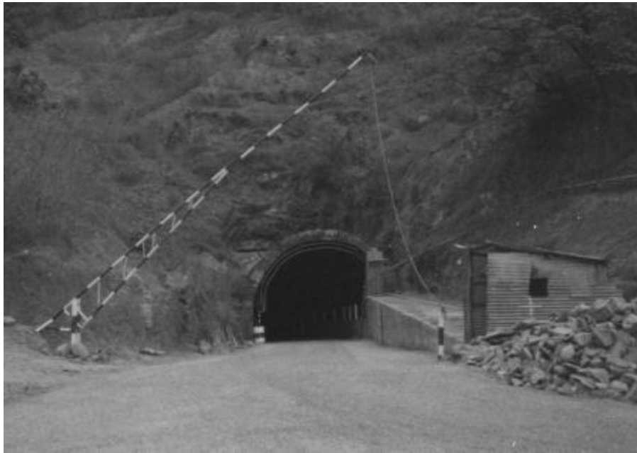
Fig. 1. Tillari HPP – entry tunnel 1986
